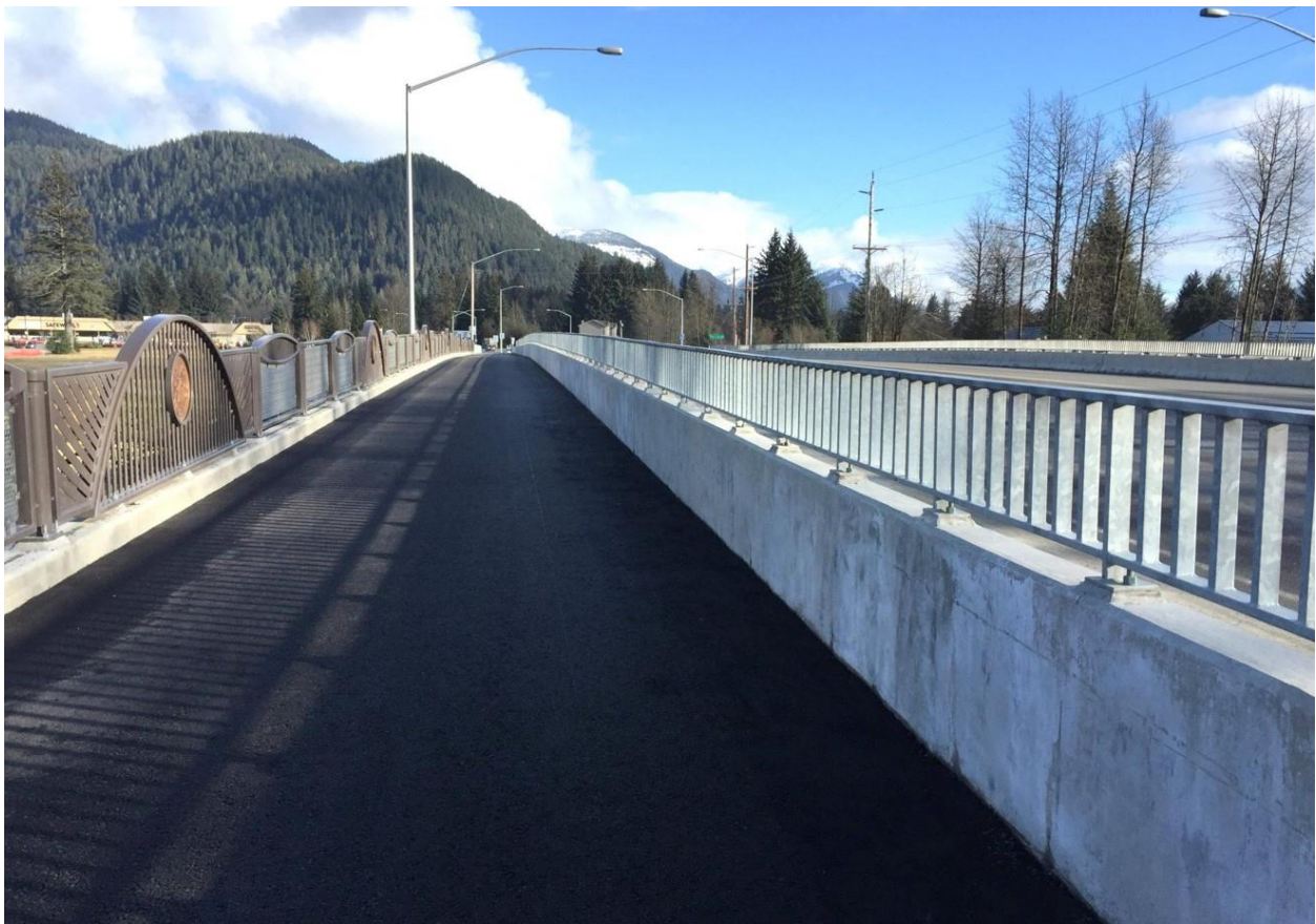
Figure 28. The bridge replacement project featured a separated path for bicycling and walking. Image courtesy of the FHWA Alaska Division Office.
