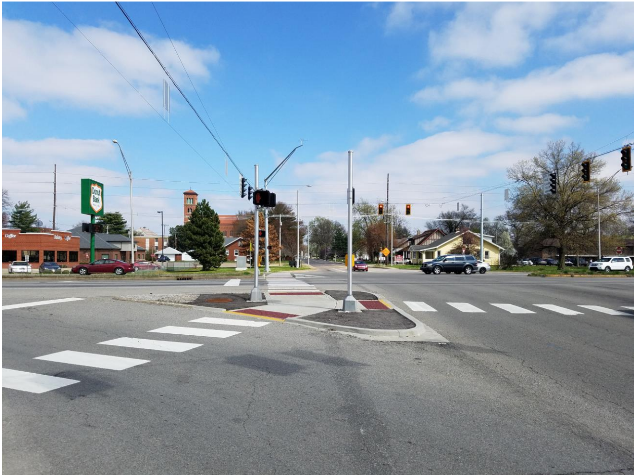
Figure 30. Islands like this one were installed to help break up long crossing distances at several intersections in Evansville, Indiana. Image courtesy of the FHWA Indiana Division Office.
