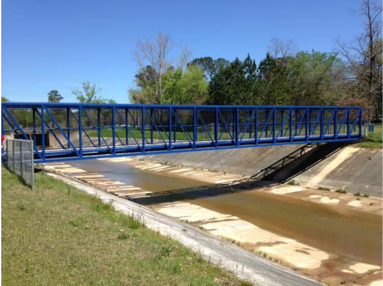
Figure 32. The new bridge over Gallagher Creek provides a critical connection for children to access the school.
