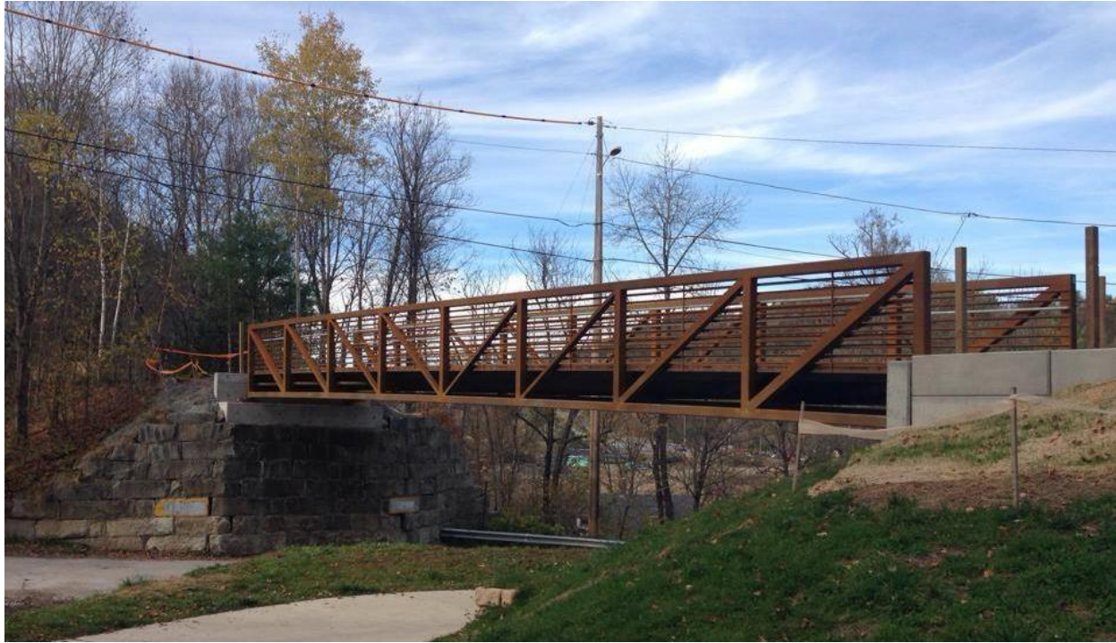
Figure 21. One of several bridges intended to improve crossings along the Lamoille Valley Rail Trail.
