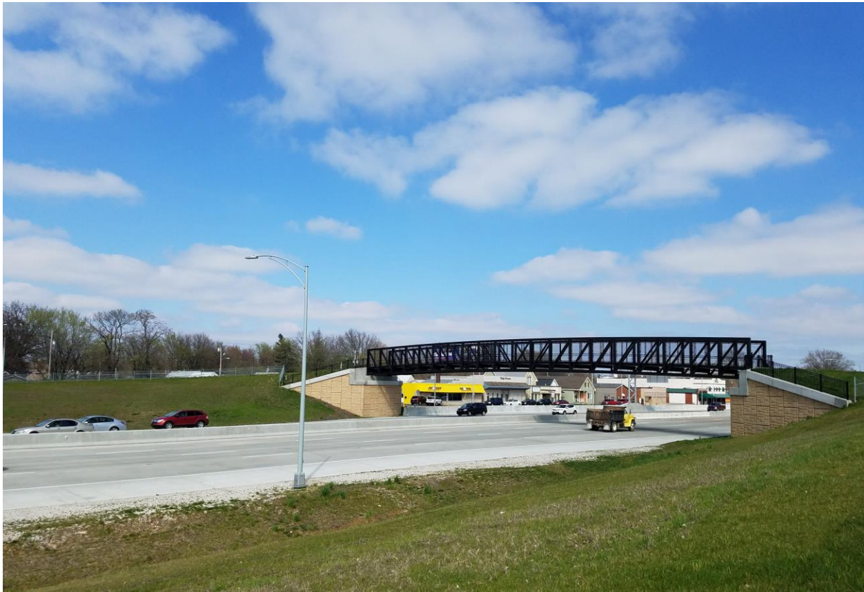
Figure 27. This bridge provides a safe way to cross Lloyd Expressway. Image courtesy of the FHWA Indiana Division Office.
