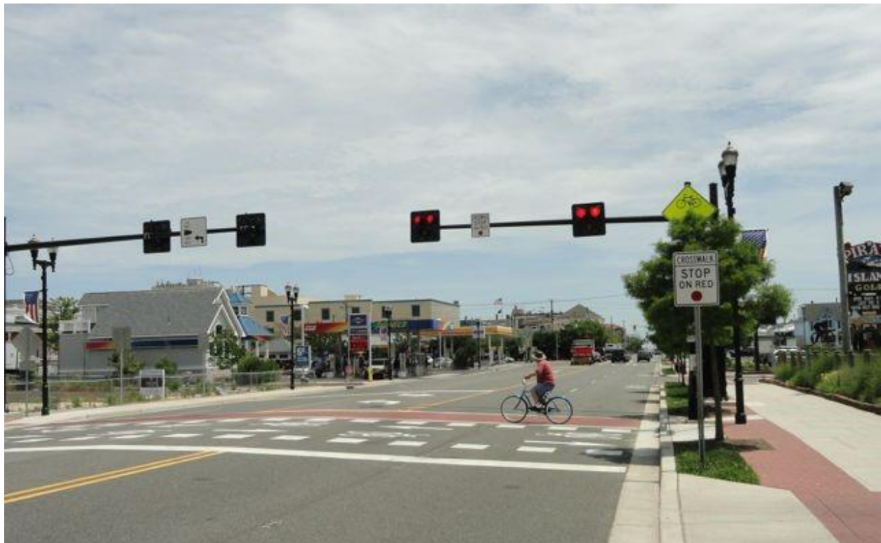
Figure 25. The Pedestrian Hybrid Beacon at 9th Street and Haven Avenue. Image courtesy of the FHWA New Jersey Division Office.
