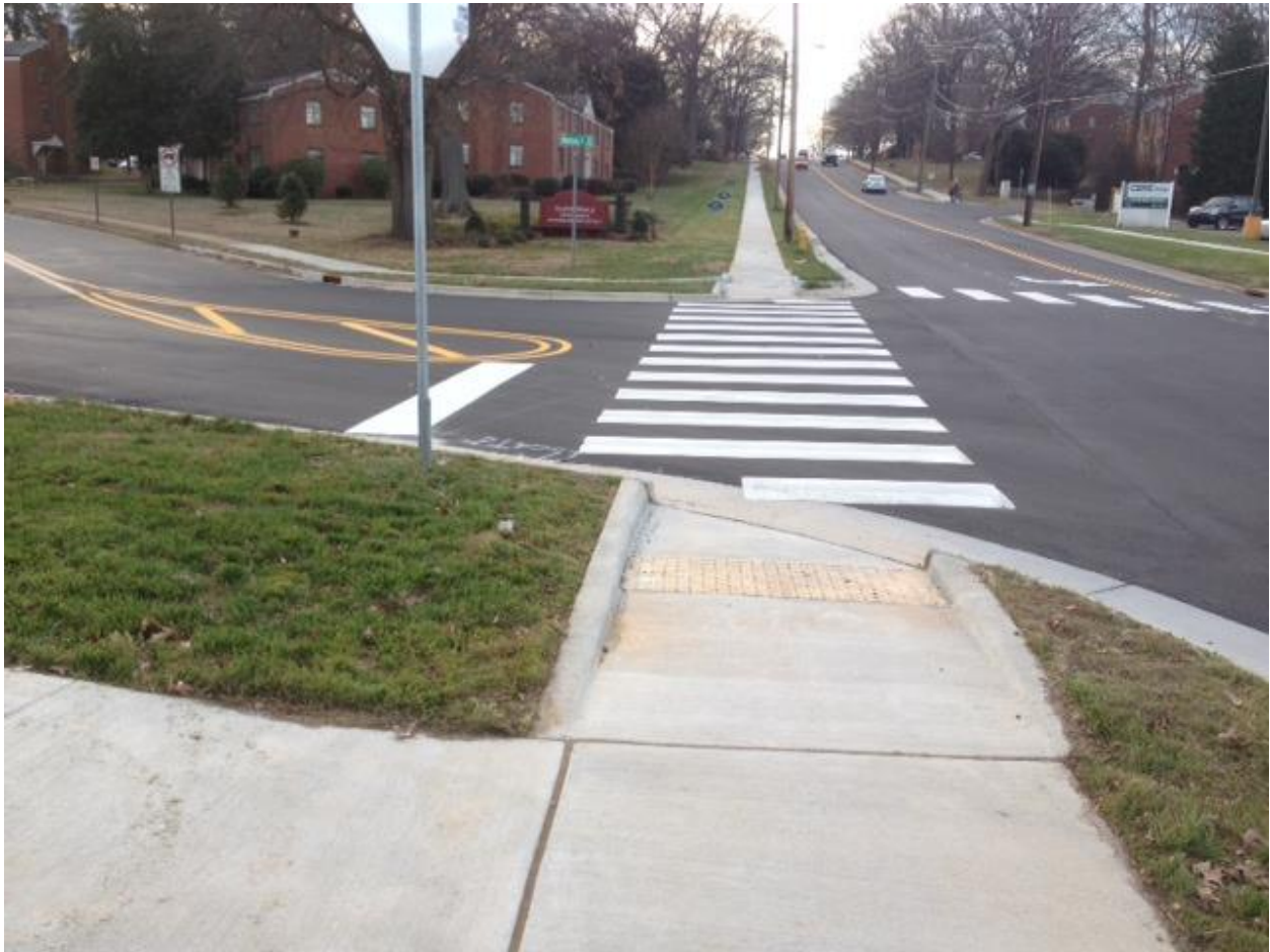
Figure 23. A realigned intersection with improved crossings was just one of the improvements along Cloverdale Avenue. Image courtesy of the City of Winston Salem.
