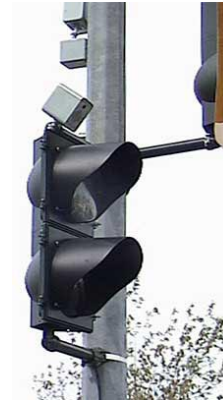
FIG. 5-3. EXAMPLE OF PEDHEAD- MOUNTED APS SPEAKER AIMED TOWARD CENTER OF CROSSWALK.
