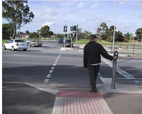
FIG. 4-8. TYPICAL APS LOCATION IN RELATION TO THE CROSSWALK AND SIDEWALK. AUSTRALIAN CURB RAMP STANDARDS ALLOW A STEEPER FLARE THAN ALLOWED BY US STANDARDS.
