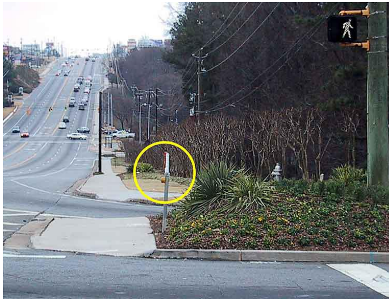
FIG. 12-15. A STUB POLE IS USED TO SITE THE PUSHBUTTON BESIDE THE SIDEWALK.
