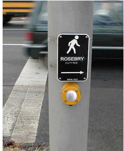
FIG. 7-7. BRAILLE LARGE PRINT STREET NAME ARE ON A SIGN ABOVE THE PUSHBUTTON.
