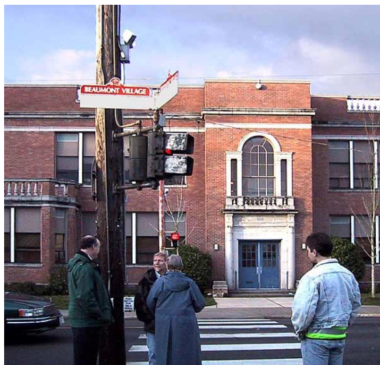
FIG. 14-3. APS MOUNTED OVER 12 FEET HIGH ON THE POLE BROADCAST SPEECH MESSAGES AT THIS LOCATION IN PORTLAND. CITY ENGINEERS EXPRESSED CONCERNS ABOUT INTELLIGIBILITY OF THE MESSAGE.
