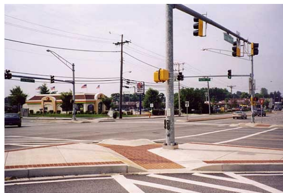
FIG. 14-13. APS AS SEEN FROM RIGHT-TURN LANE CROSSING.
