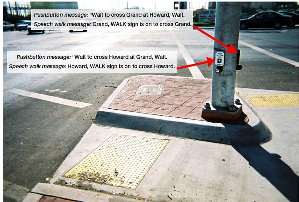
FIG. 11-5. EXAMPLE OF PUSHBUTTON INFORMATION MESSAGES AND SPEECH WALK MESSAGES FOR TWO APS LOCATED ON THE SAME POLE
