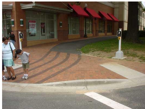
FIG. 14-1. (LEFT) PUSHBUTTON-INTEGRATED APS LOCATED ON A STUB POLE BESIDE THE LEVEL LANDING OF THE CURB RAMP.
