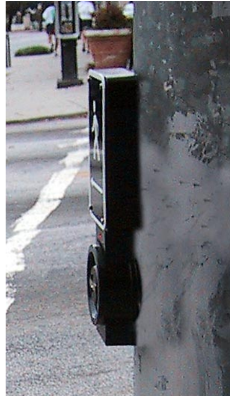
FIG. 12-12. TYPICAL INSTALLATION WITHOUT EXTRA MOUNTING PLATE, WITH WIRE RUNNING FROM INSIDE METAL POLE INTO THE BACK OF THE DEVICE.
