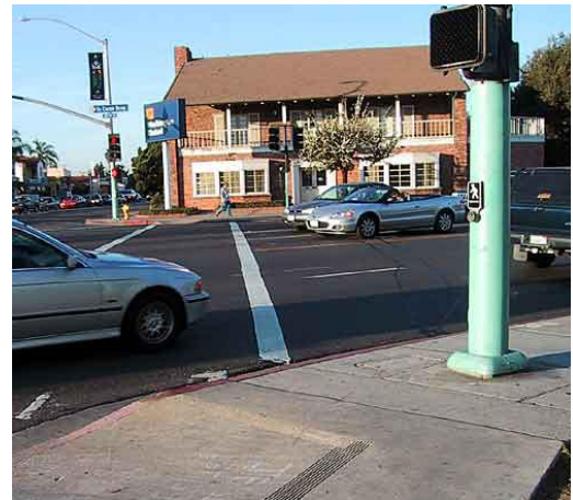
FIG. 12-31. IN A SIMILAR SITUATION, THIS PEDESTRIAN SIGNAL HEAD FOR THE E/W CROSSWALK IS DIRECTLY OVER THE WAITING LOCATION FOR THE N/S CROSSWALK, HOWEVER IN THIS INSTANCE THE APS MOUNTED ON THAT PEDHEAD IS PROPERLY WIRED TO SOUND FOR THE N/S CROSSWALK.
