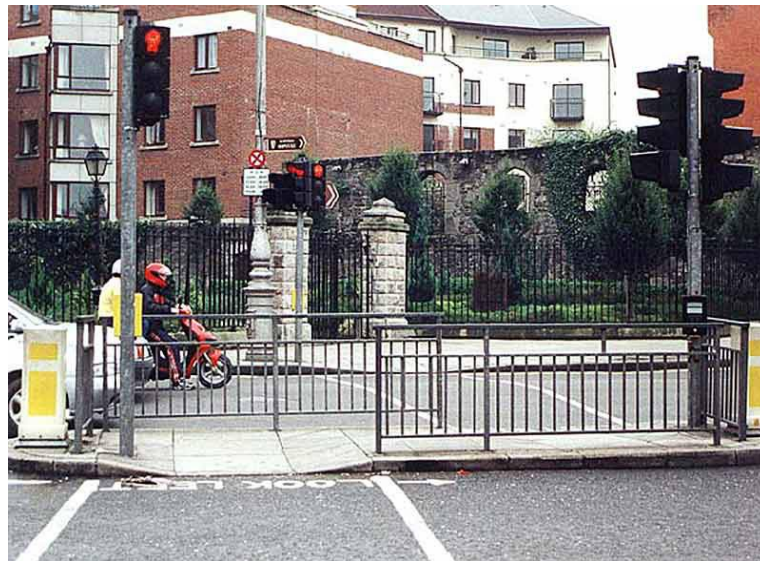
FIG. 9-1. AT THIS MEDIAN ISLAND IN IRELAND, AN APS IS PROVIDED FOR EACH CROSSING, A FENCE PREVENTS PEDESTRIANS FROM CONTINUING STRAIGHT ACROSS THE STREET, REQUIRING THE PEDES- TRIAN TO TURN AND WALK TO THE OTHER CROSSWALK LOCATION AND PUSHBUTTON.
