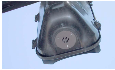
FIG. 4-4. JAPANESE PEDHEAD WITH APS SPEAKER POINTING STRAIGHT DOWN TOWARD THE PEDESTRIAN BELOW.
