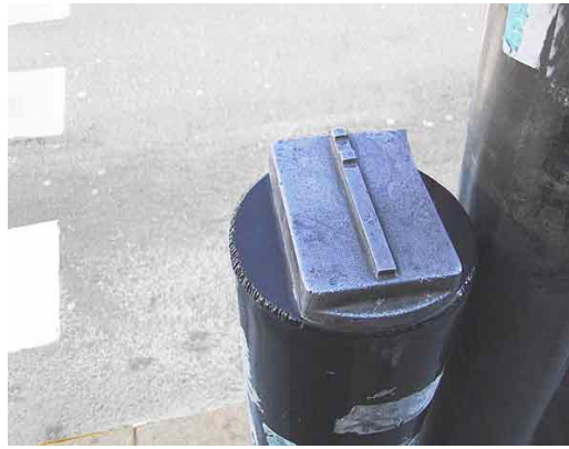
FIG. 4-16. DANISH APS WITH TACTILE BAR MOUNTED ON THE TOP. THE BAR IS ALIGNED WITH THE CROSSWALK, AND TWO KNOBS AT THE END OF THE BAR INDICATE A MEDIAN AND THE FAR SIDE OF THE STREET.
