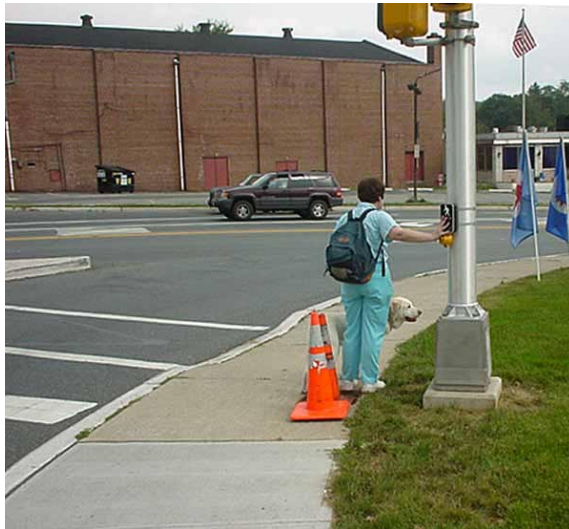
FIG. 14-9: APS MOUNTED ON SIGNAL POLE FOR CROSSING SIGNALIZED RIGHT TURN LANE. PEDESTRIAN WHO IS BLIND IS WAITING WITH HER HAND ON THE PUSHBUTTON FOR THE VIBROTACTILE WALK INDICATION. AFTER THE WALK INDICATION BEGINS, SHE MUST TURN, AND CROSS THE SIDEWALK BEFORE BEGINNING TO CROSS THE STREET.
