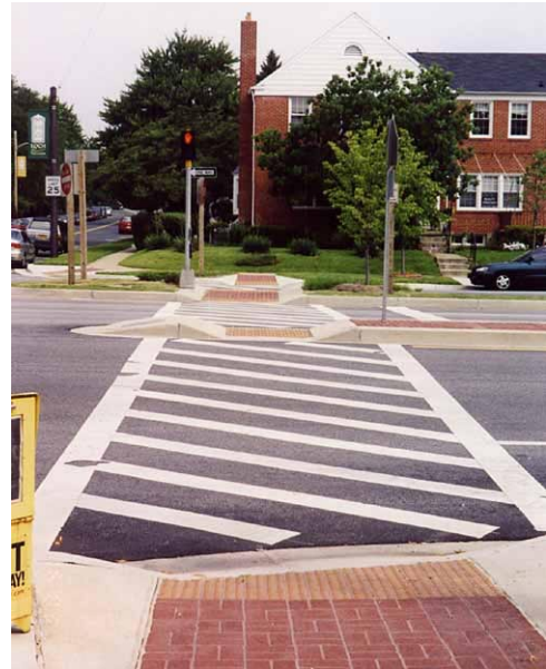
FIG. 14-15: [ABOVE] VIEW ACROSS LOCH RAVEN TOWARD TWO MEDIAN ISLANDS AND STOP SIGN CONTROLLED SERVICE ROAD.
