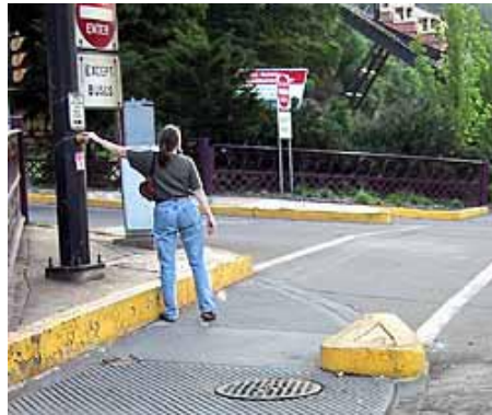
FIG. 12-4. THIS PUSHBUTTON MAY BE 42 INCHES FROM THE BOTTOM OF THE POLE, BUT IT IS ALMOST 60 INCHES ABOVE THE LANDING, NOT ACCESSIBLE TO A WHEELCHAIR USER AND NOT LIKELY TO BE LOCATED BY A PERSON WHO IS BLIND.
