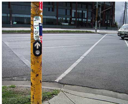
FIG. 4-9. INSTALLATION OF TACTILE ARROWS WAS NOT CONSISTENT AND PROVIDED MISLEADING INFORMATION IN SOME CASES.
