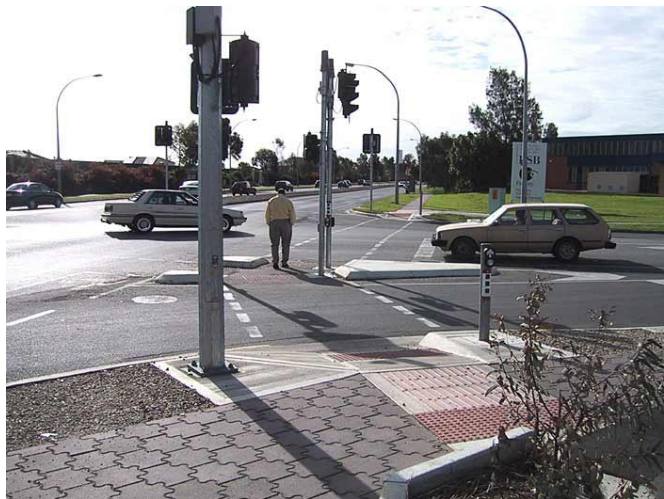
FIG. 4-6. SIGNALIZED LEFT TURN LANE WITH APS MOUNTED CLOSE TO THE CROSSWALK LOCATIONS. THREE APS ARE ON THE SPLITTER ISLAND, ONE FOR EACH CROSSING.
