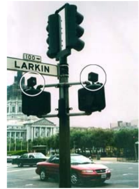
Fig. 15-15. PEDHEAD-MOUNTED APS UNITS TRANSMIT SPEECH MESSAGES TO A HANDHELD RECEIVER.
