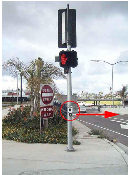
FIG. 12-30. THE PEDHEAD FOR THE N/S CROSSWALK IS LOCATED OVER THE PUSHBUTTON FOR THE E/W CROSSWALK. THE SPEAKER LOCATED ON THE SIDE OF THE PEDHEAD, AND DIRECTLY OVER THE WAITING AREA TO CROSS E/W, SOUNDS FOR THE N/S CROSSWALK. IT IS VERY EASY TO BE CONFUSED, SINCE THE SOUND FOR THE E/W CROSSWALK IS LOCATED DIRECTLY ABOVE THE N/S CROSSWALK WAITING AREA.
