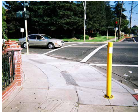
FIG. 11-3. APS ARE POSITIONED APPROPRIATELY AT THIS INTERSECTION BY THE ADDITION OF A STUB POLE FOR ONE CROSSWALK. THE STUB POLE HOLDING THE APS FOR THE CROSSWALK AT RIGHT IS SIMPLY BOLTED IN. THE OTHER APS IS MOUNTED ON THE POLE THAT SUPPORTS THE PEDHEAD.
