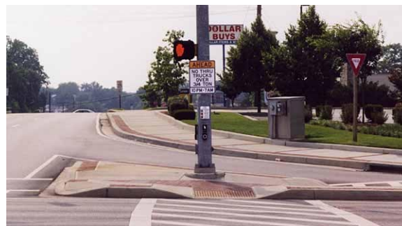
FIG. 14-12. TWO APS ARE MOUNTED ON THE EXISTING POLE ON THIS ISLAND.
