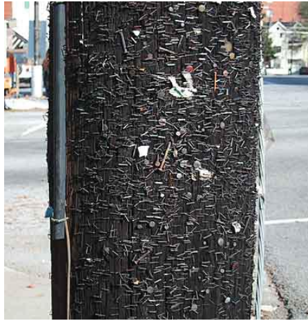
FIG. 12-13. WOODEN POLE WITH NAILS AND STAPLES THAT ARE TYPICAL AND SOURCE OF CONCERN.
