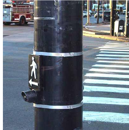
FIG. 12-9. POORLY LOCATED APS ON A ROUND POLE POINTS INTO THE INTERSECTION.
