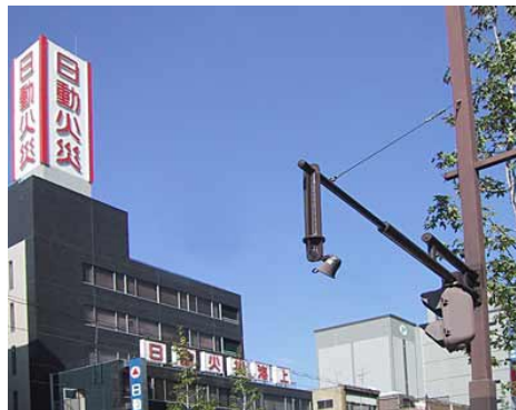
FIG. 4-3. PEDHEAD WITH APS SPEAKER IS MOUNTED ON A MAST ARM OVERHANGING THE CROSSWALK BELOW.
