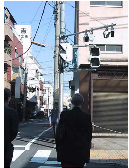
FIG. 4-5. THE PICS-A SYSTEM IS SHOWN WITH FOUR INFRARED TRANSMITTERS MOUNTED ON A HORIZONTAL MAST ARM
