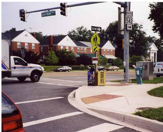
FIG. 14-16. APS INSTALLED ON SIGNAL POLE BESIDE CROSSWALK WAITING LOCATION.
