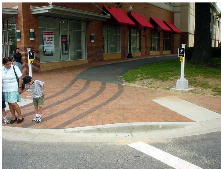
FIG. 10-6. APS INSTALLED IN THIS RECONSTRUCTION LOCATION IN ACCORD- ANCE WITH THE DRAFT GUIDELINES BESIDE A LEVEL LANDING, WITHIN 5 FEET OF THE CROSS- WALK LINE EXTENDED AND LESS THAN 10 FEET FROM THE CURB. THE CONTROL FACES AND PUSHBUTTONS FACE THE INTERSECTION.
