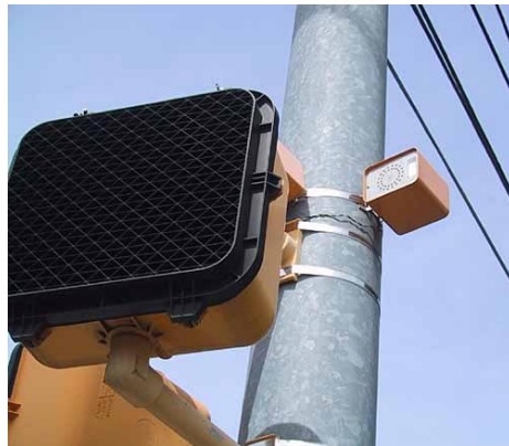
FIG. 14-19. PEDHEAD-MOUNTED SPEAKER MOUNTED ON THE POLE AS TYPICALLY INSTALLED IN ATLANTA.
