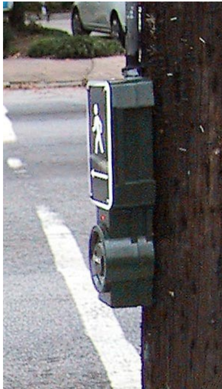
FIG. 12-11. MOUNTED ON THE WOODEN POLE, AN ADDITIONAL MOUNTING BRACKET IS INSTALLED TO ALLOW THE WIRES TO RUN FROM CONDUIT INTO THE TOP OF THE PUSHBUTTON-INTEGRATED DEVICE.
