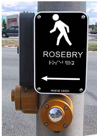
FIG. 12-18. BRAILLE LABEL IS BELOW THE RAISED PRINT STREET NAME.
