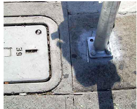
FIG. 12-17. STUB POLE INSTALLED NEAR SIDEWALK SIGNAL BOX SIMPLIFIES WIRING AND LOCATES PED PUSHBUTTON BY THE CROSSWALK.
