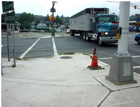
FIG. 14-8. INSTALLATION OF TWO PUSHBUTTONS ON A SINGLE POLE (ONLY A SINGLE PUSH-BUTTON IS VISIBLE IN THE PHOTO). WHILE THE PUSH-BUTTON IS IN LINE WITH THE CROSSWALK, THE PEDESTRIAN MUST TRAVEL OVER 10 FEET BEFORE REACHING THE STREET AND THE BEGINNING OF THE CROSSWALK.
