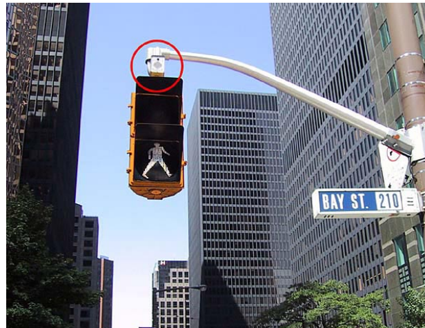
FIG. 11-1. MAST ARM IS USED IN THIS INSTALLATION IN TORONTO, CANADA TO POSITION PEDESTRIAN SIGNAL HEAD AND SPEAKER CLOSER TO THE CROSSWALK.
