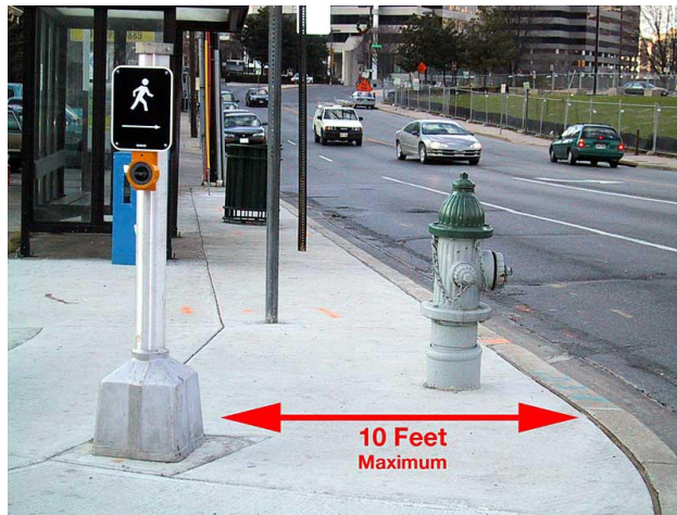
FIG. 10-5. THE APS SHOULD BE WITHIN 10 FEET OF THE CURB
