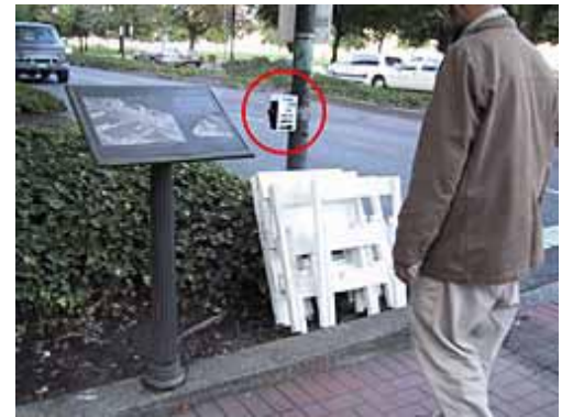
FIG. 12-5. NOT ONLY IS THE PUSHBUTTON IN THE BUSHES, CONSTRUCTION BARRIERS HAVE BEEN STORED AGAINST THE POLE, PREVENTING PEDESTRIANS FROM REACHING THE PUSHBUTTONS.
