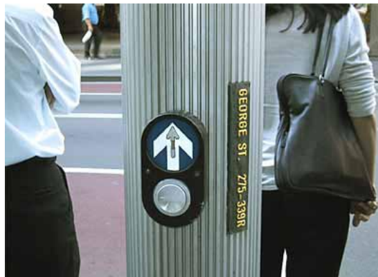
FIG. 7-8. A RAISED PRINT AND BRAILLE SIGN IS MOUNTED VERTICALLY ON A ROUND POLE TO THE RIGHT OF AN APS. THE SIGN READS "GEORGE ST. 275-339R".
