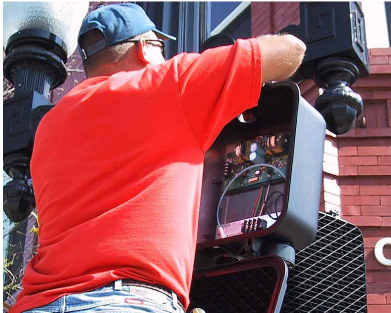
FIG. 12-1. INSTALLER POSITIONING THE APS CONTROLLER BOARD INSIDE THE BACK OF THE PEDESTRIAN SIGNAL HEAD.
