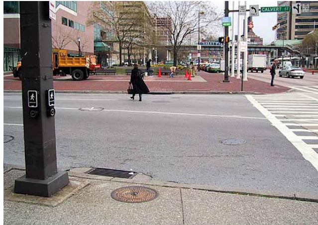
FIG. 12-6. IF PEDESTRIANS PROCEED DIRECTLY TO THE CURB FROM THE PUSHBUTTON IN THIS PHOTO, THEY WILL BE WELL OUTSIDE THE CROSSWALK AREA WHEN BEGINNING THEIR CROSSING.
