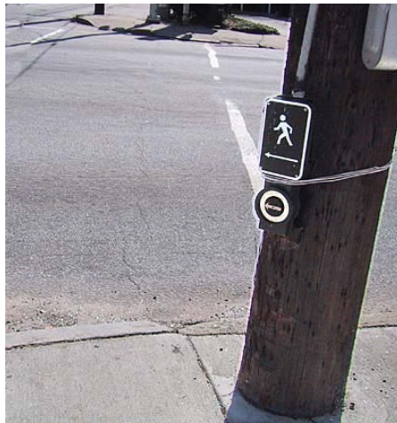
FIGURE 13-2: APS WAS REPLACED ON THE POLE, BUT THE TACTILE ARROW POINTS TO THE CENTER OF THE INTERSECTION, RATHER THAN BEING ALIGNED WITH THE DIRECTION OF TRAVEL ON THE CROSSWALK.
