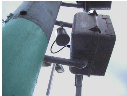
FIG. 5-2. EXAMPLE OF PEDHEAD- MOUNTED APS SPEAKER AIMED AT PEDESTRIAN WAITING LOCATION.
