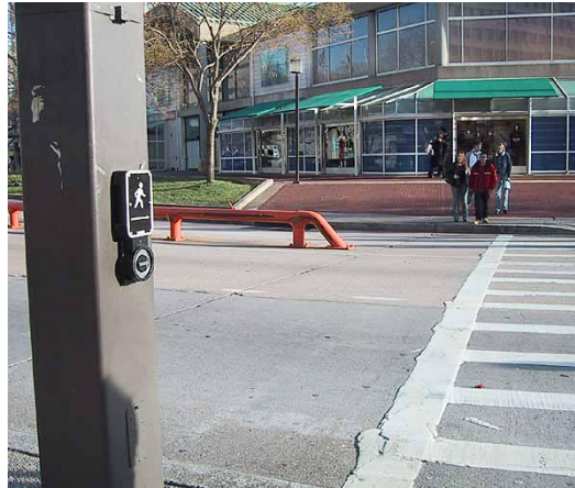
FIG. 12-8. WELL LOCATED APS ON A SQUARE POLE.
