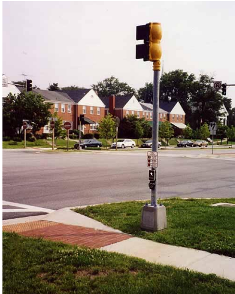
FIG. 14-14 APS INSTALLED ON PEDESTRIAN SIGNAL POLE
