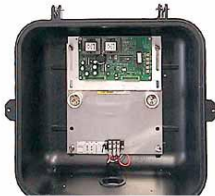
FIG. 12-2. CONTROLLER BOARD MOUNTED BEHIND 18 INCH PEDESTRIAN SIGNAL HEAD.
