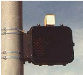
FIG. 5-1. APS UNIT MOUNTED ON TOP OF PEDHEAD.
