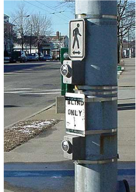
FIG. 7-9. CONTRARY TO PROWAAC RECOMMENDATIONS, THE PHOTO SHOWS AN ADDITIONAL BUTTON USED TO BRING UP ADDITIONAL ACCESSIBLE FEATURES. THE LOWER SIGN READS “BLIND ONLY.”
