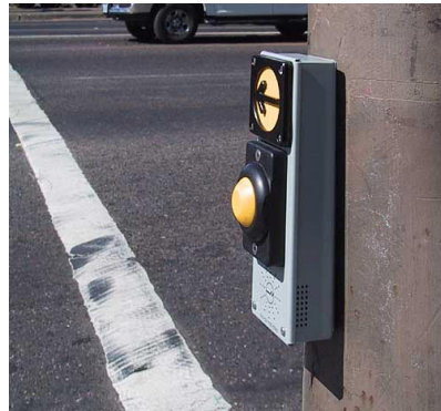
FIG. 14-4. VIBRAWALK PUSHBUTTON INSTALLED IN PORTLAND INCLUDES A LOCATOR TONE. THE ARROW VIBRATES DURING THE WALK INTERVAL AND WALK INDICATION IS PROVIDED FROM PUSHBUTTON OR SPEAKER MOUNTED ON THE PEDHEAD.
