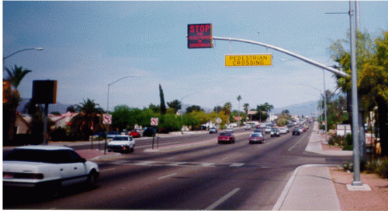
Figure 12. The installation of the pedestrian regulatory signs on four- and six-lane arterial roads in Tucson may have limited their effectiveness.
