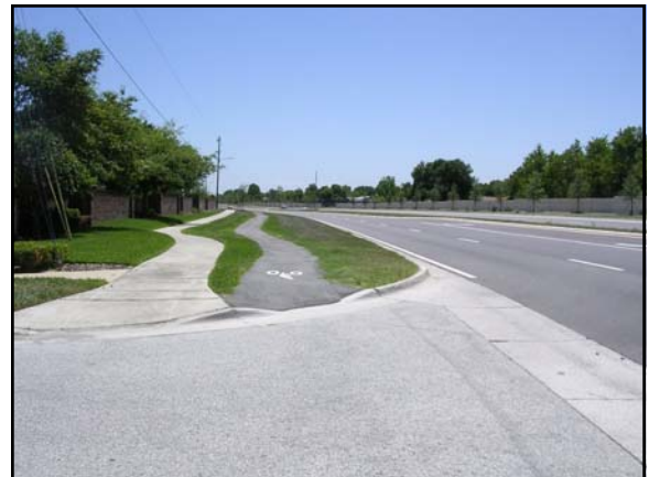
Unidirectional Bicycle Path on Apopka-Vineland Road, Orange County
