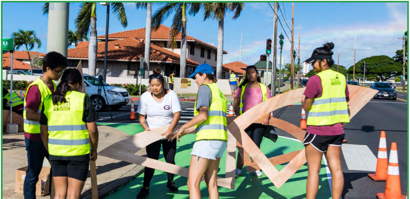
Youth and adults working on a quick-build installation. Source: Ulupono Initiative
