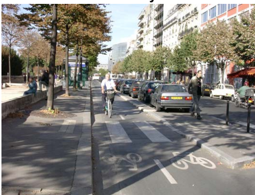
Figure 11. Physically Separated Bi-Directional Bicycle Lane
