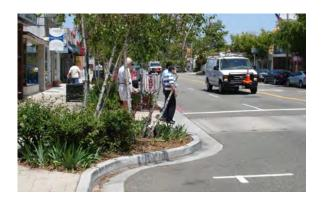
**Bulb-outs or curb extensions** – Bulb-outs shorten the distance trail users need to cross and improve visibility of trail users for approaching vehicles. They can be used in areas where street parking is allowed or in a shoulder if they will not impede bike flow. Bulb-outs can also help reduce traffic speeds as they narrow the roadway and field of vision for drivers. The design should avoid encroachment into the travel lane that would create a pinch point
