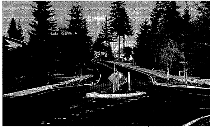
Traffic Circle or Roundabout with Curb Extensions
