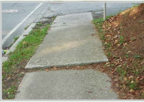
Hazardous sidewalk discontinuity
