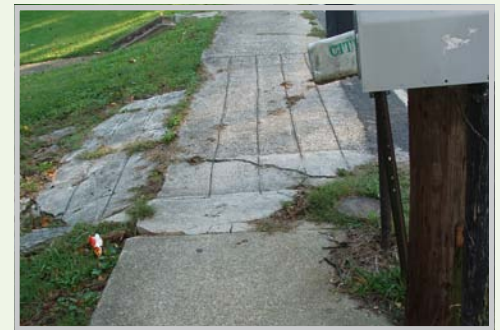
Unsafe driveway crossing
