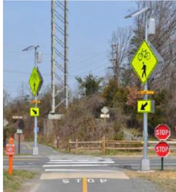
Rectangular Rapid Flashing Beacon
