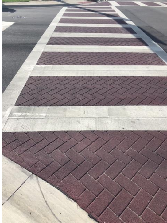
High Visibility Crosswalks Hillsboro Blvd. City of Deerfield Beach
