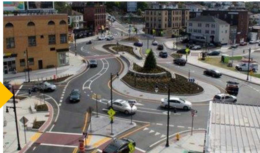
Newly built Kelley Square, Worcester
