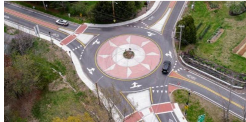
New roundabout on Route 140, Princeton, MA
