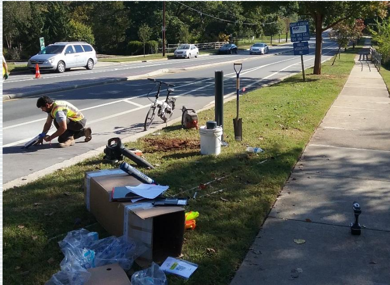
At new station installation
