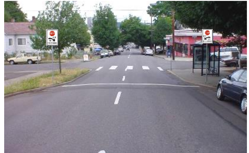
Advance stop line and sign
