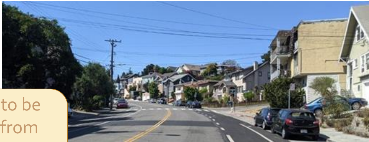
HVC Marking on Driver Approach (approximately 150 feet upstream).
