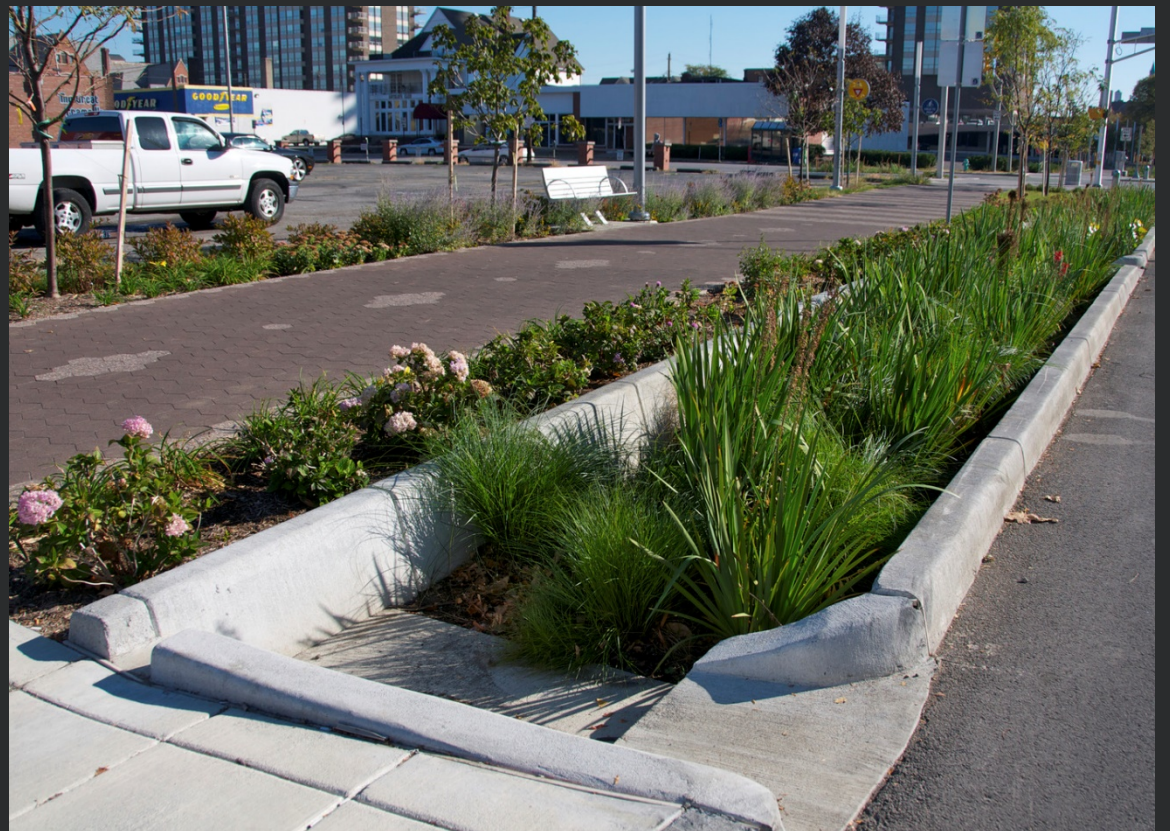
Green Infrastructure on the Indianapolis Cultural Trail Image: Toole Design
