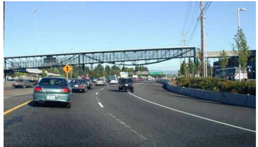
Light rail stations
