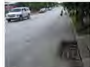
Below-grade drain grates create hazards for bicyclists.
