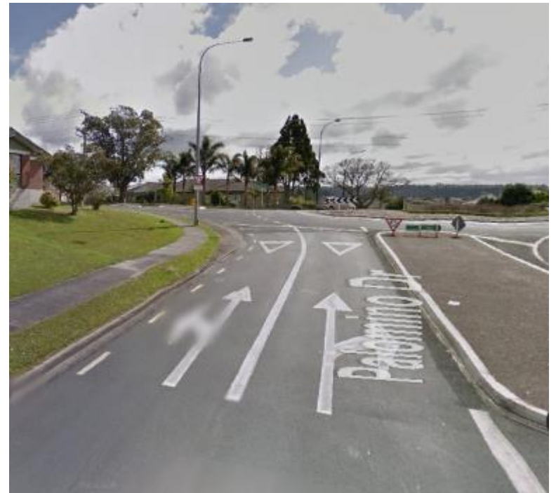
C-Roundabout. (Source: © Google, 2015. Image, 2012)
