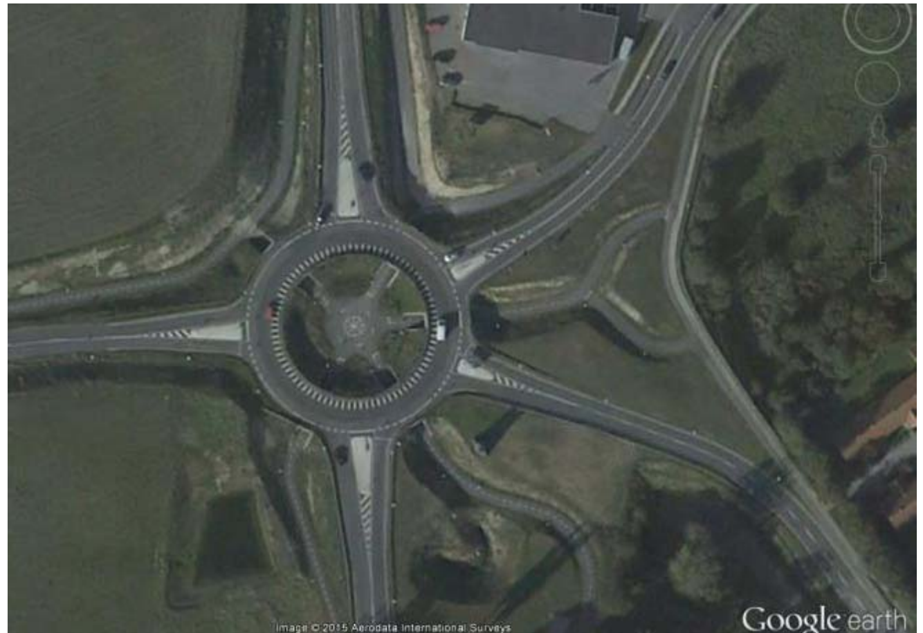
Shared Use Path Grade Separations, Haderslev, Denmark (Source: 2015 Google et al.)
