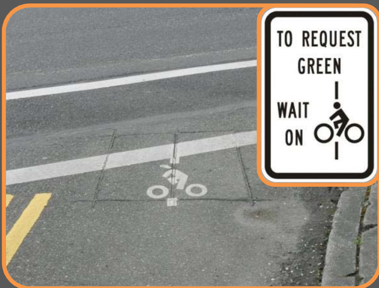
Pavement Markings & Signing for Loop Detectors
