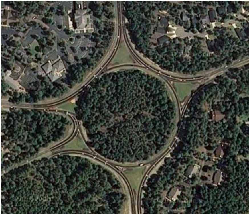
(Large) Traffic Circle, Pinehurst, NC
