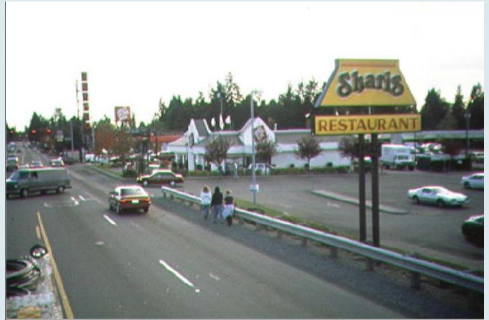
Bridgeport Way, prior to improvements
