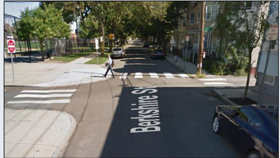
Curb Extension at Berkshire St & York St
