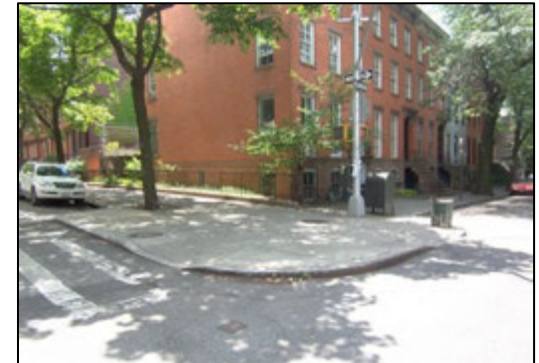
Sidewalk Extensions: Shortens crossing distance, slows turning cars
