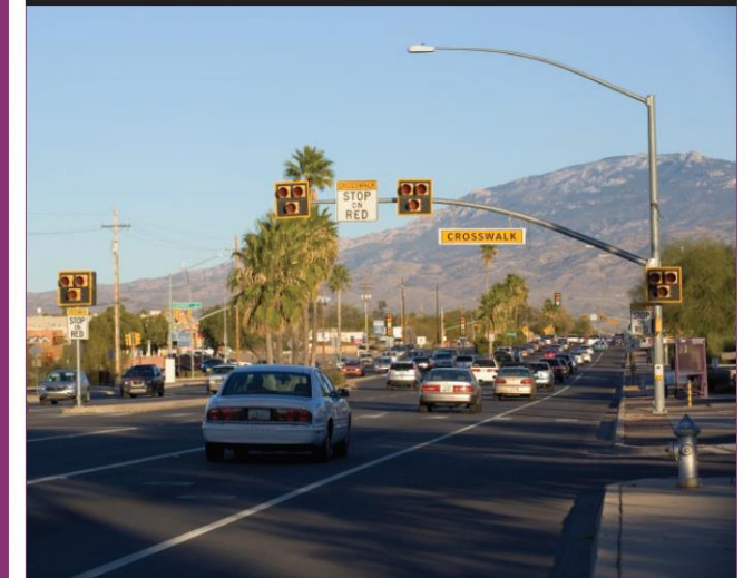
Figure 1. Example of PHB installation in Tucson, AZ.
