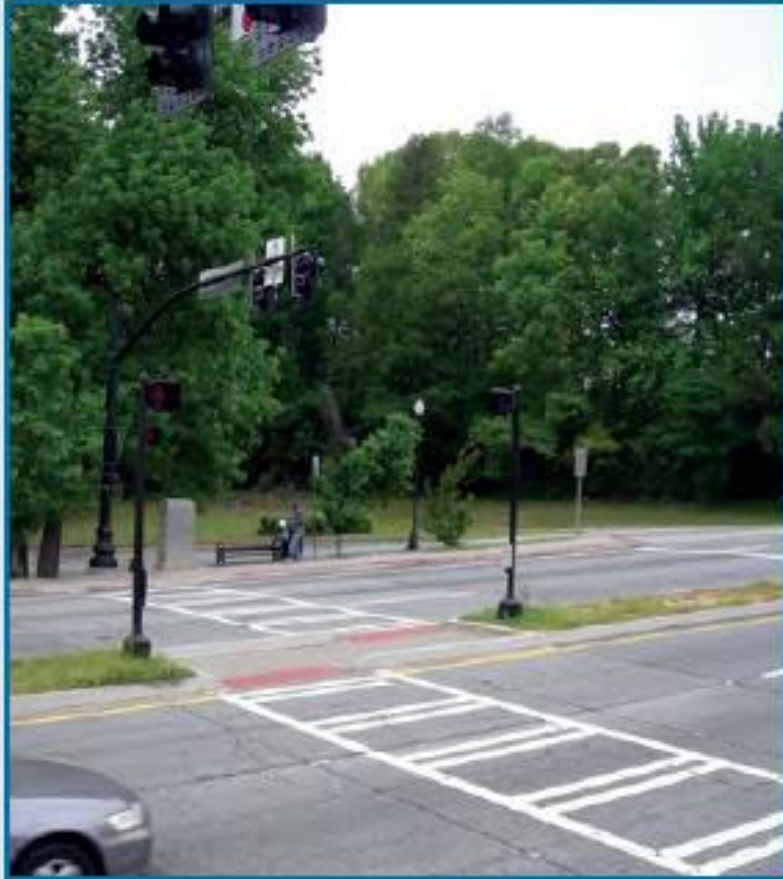
Figure 7. PHB installed on Buford Highway near pedestrian attractors: a transit stop. Photo credit: Bruce Landis
