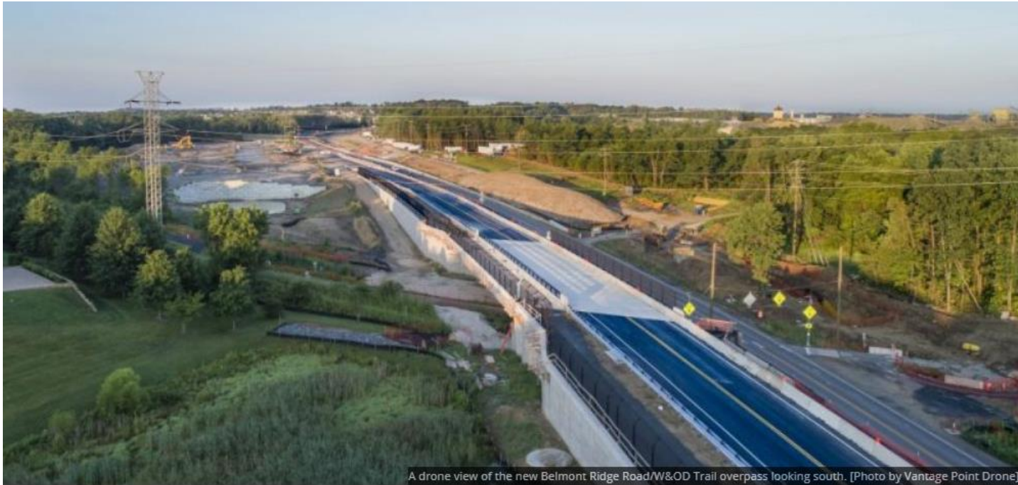
A drone view of the new Belmont Ridge Road/W&OD Trail overpass looking south. [Photo by Vantage Point Drone]
