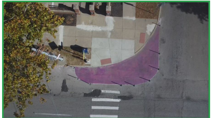
A drone image of a curb extension at the intersection of Linn Street and Chestnut Street in Cincinnati. Source: Christian Hauser.
