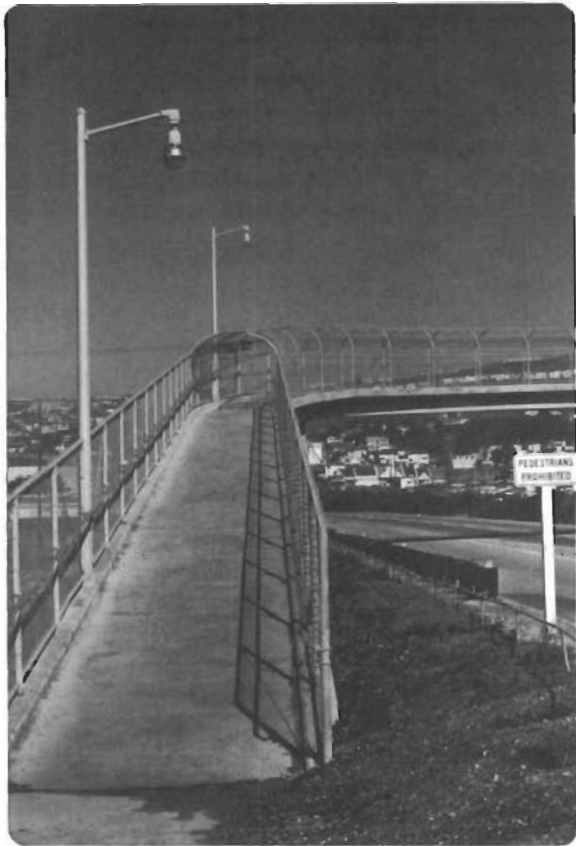
A major bikeway grade separation structure.
