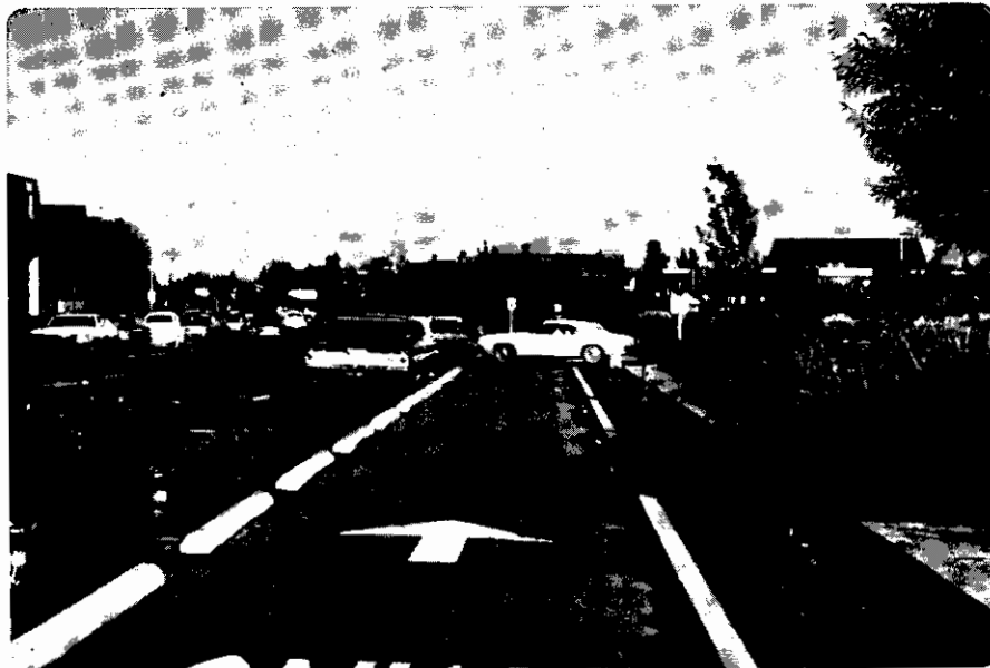
Figure 4: TYPICAL PROTECTED LANE (Davis, California) NOTE USE OF CONCRETE "PARKING LOT BUMPER BLOCKS" AS BARRIER
