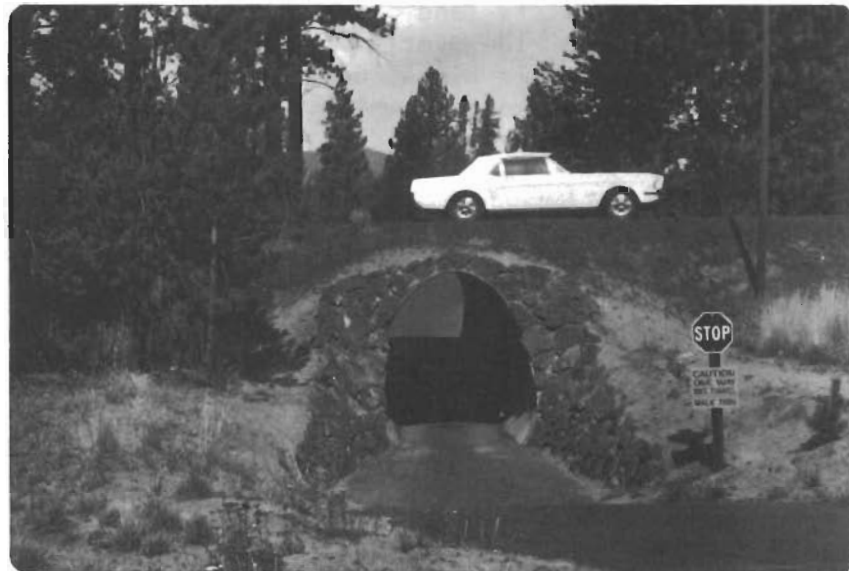
A simple bikeway grade separation of corrugated pipe. Note minimized adverse grade profile on bikeway made possible by elevation of roadway and use of underpass.
