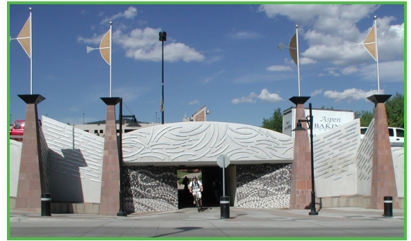
A new pedestrian and bicycle tunnel along 28th Street.
