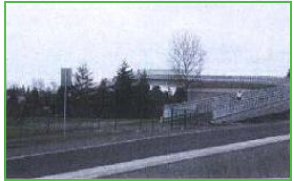
The ramp leading up to the bridge.
