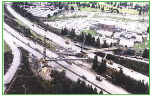
Aerial view of the bridge during construction.
