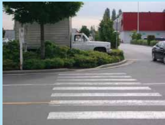
An absence of continuity is apparent in this photograph, where a marked pedestrian crosswalk over a circulating road in a commercial development ends in a landscaped area. No connecting walkway is provided, so pedestrians must walk in the street.
