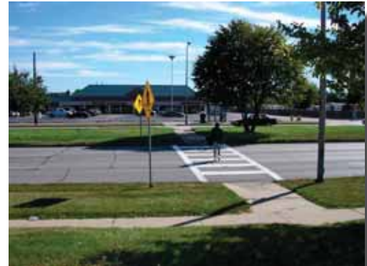
The raised median above is accessible to all pedestrians and provides a large waiting area.
