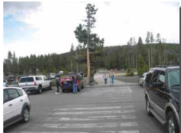
Vehicles in pull-in parking stalls immediately adjacent to a marked crosswalk obstruct sightlines between circulating vehicles and pedestrians in and approaching the crosswalk. The obstruction is transient, since sightlines would improve when the stalls are unoccupied. In addition to obstructing sightlines, vehicles backing out of the stalls may conflict with pedestrians in the crosswalk.
