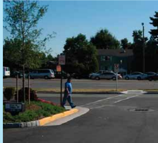
This shopping facility has a frontage road parallel to a busy, arterial highway. Pedestrian facilities and signage creates a circuitous route, which does not follow pedestrian desire lines and puts pedestrians in conflict with traffic on the frontage road. As is seen in this photograph, pedestrians will often ignore the pedestrian facilities and walk instead in the frontage road closer to the commercial establishments.
