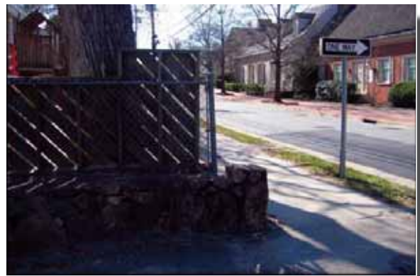
A motorist backing out of the driveway would have a difficult time viewing pedestrians walking on the sidewalk.
