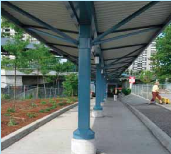
A covered walkway has been provided to connect a major shopping center and transit station, but the walkway does not follow pedestrian desire lines. As a result, pedestrians frequently shortcut through the shopping center parking lot (as shown in the photograph), where no designated pedestrian pathway is available.
