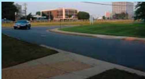
The crossing is positioned beyond a horizontal curve. Drivers such as the one in the photo are unlikely to see the crossing (which is not marked by signs or pavement markings) until they are exiting the curve, at which point drivers are typically accelerating. The curve also limits the distance at which headlights would illuminate the crossing, so the risk of a pedestrian crash is increased at night. Also, a pedestrian crossing toward the camera is facing away from vehicles approaching around the curve, and may consequently be less aware of them. Finally, the curb ramps are offset, increasing exposure of pedestrians and increasing the difficulty of the crossing for someone with visual limitations. The RSA team may suggest moving this crossing away from the curve and place the curb ramps directly across from each other.
