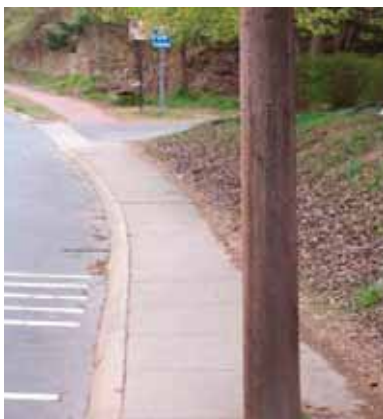
The photo on the left shows access to a bus stop (in the distance) obstructed by a telephone pole. Access to the bus shelter on the right is inhibited due to a missing connection between the sidewalk and the bus shelter landing.
