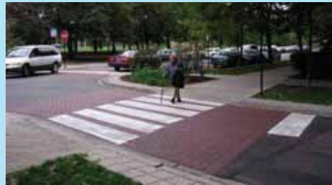
The curb radii at the intersection in this photo are small, minimizing the crosswalk length and reducing pedestrian exposure to vehicular traffic. This residential street, with young and elderly pedestrians, is a good location for short curb radii. Access for emergency vehicles has been maintained by utilizing a low curb profile on the corners with pavers, which allows emergency vehicles to mount the curb.
