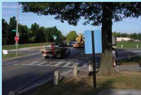
In the intersection shown above, a tree partially obstructs the view of pedestrians waiting to cross the street. Motorists approaching this intersection to turn right focus their attention on finding a gap in traffic by looking for approaching conflicting vehicles to their left.
