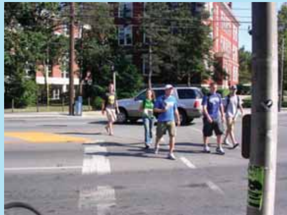
The narrow crosswalk likely meets minimum requirements for crosswalk width, but cannot accommodate three pedestrians walking abreast. The crosswalk markings should align with the ramp at the far side of the intersection, so that pedestrians entering the roadway from the ramp are within the crosswalk markings. The RSA team may suggest applying high-visibility crosswalk markings of sufficient width to accommodate pedestrian volumes.
