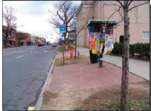
A landing area with significant slopes in any direction is a safety concern, especially for people with disabilities or using strollers.
