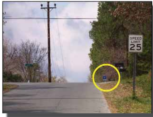
Pedestrians crossing the street to reach the bus stop circled in the photograph above will be hidden by the crest of the vertical curve.
