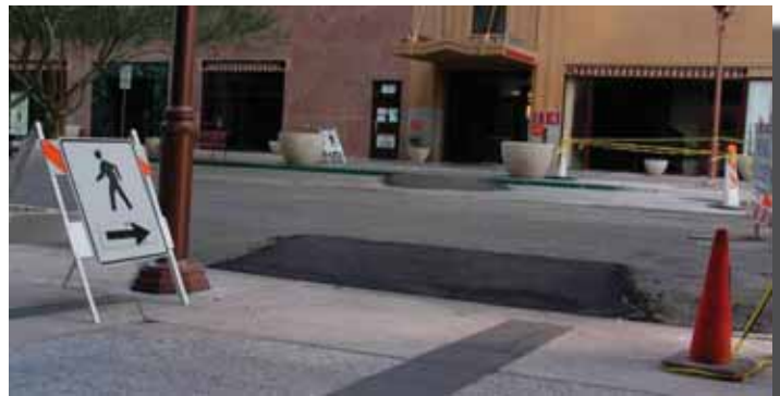
A good example of a temporary curb ramp is one made of a stable material such as asphalt or concrete, not sand or wood.
