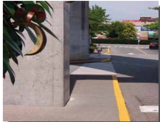
Large columns obstruct sightlines between pedestrians approaching marked crosswalks and vehicles exiting a parking area. The columns also limit the sidewalk width.
