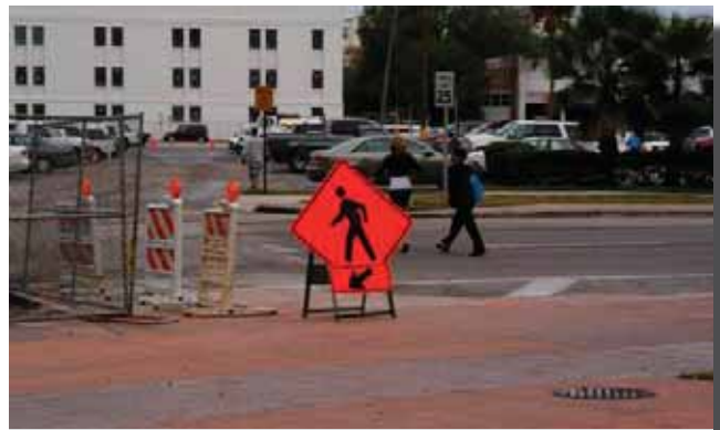
Inappropriate signage and channelization fails to effectively convey safe travel paths for pedestrians. In the photo above, the wrong signing fails to direct pedestrians to the proper crossing.
