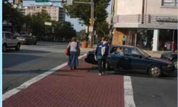
The two photos show a vehicle making a permissive left turn in front of oncoming traffic and nearly hitting pedestrians in a crosswalk during the WALK interval. The RSA team may suggest providing a protected left turn that does not conflict with the pedestrian WALK interval.
