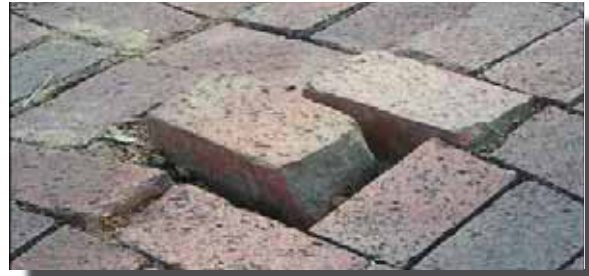
Brick sidewalks can be susceptible to changes in level.
