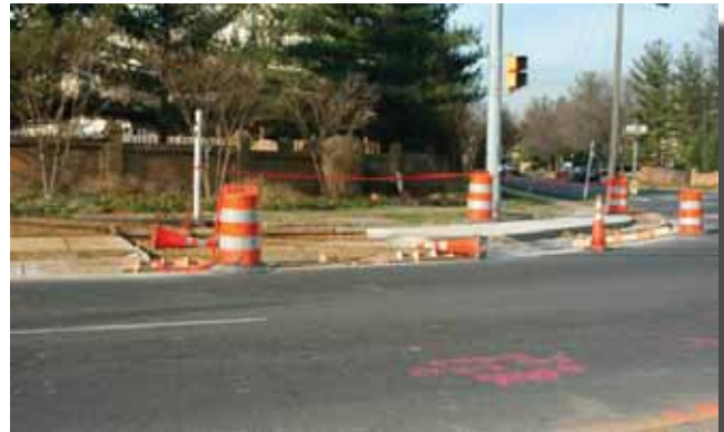
Pedestrian paths should be continuous, even during periods of construction. In the photo above, an alternate accessible path around construction has not been provided, leaving a gap in the sidewalk.
