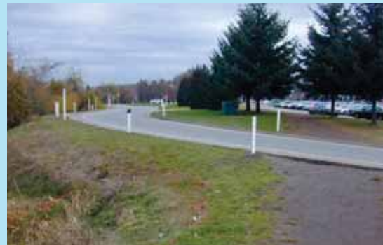
Pedestrian facilities should be provided to accommodate pedestrian demand and desire lines. In this photograph, pedestrians have worn a direct path between a parking area and a large pedestrian generator. No roadway crossing facilities are provided for this “unofficial” pathway, with the result that pedestrians using it must cross an unlighted, curved interchange ramp access where drivers may not expect pedestrians.
