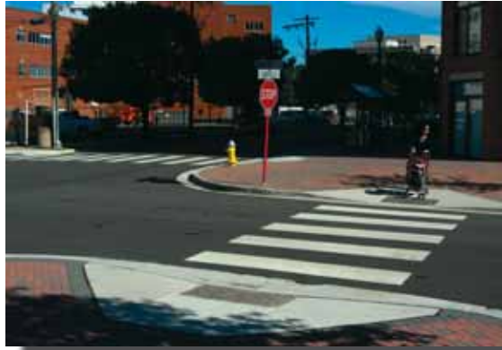
Curb ramps and cut throughs are oriented directly in line with the crosswalks, so that pedestrians do not need to walk outside the crosswalk markings when entering or leaving the crosswalk. The ramps correctly orient pedestrians with low vision along the crosswalk alignment when they are entering the crosswalk.
