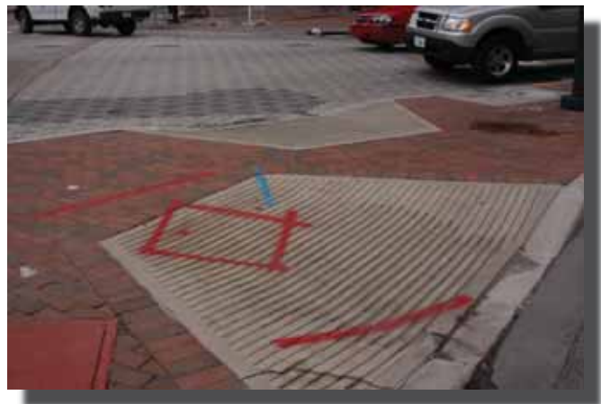
The level landings for each of these ramps on this refuge island do not connect, making it difficult for pedestrians with vision or mobility restrictions.
