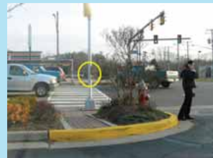
A well-marked crosswalk (far side) ends at a sidewalk that is partly obstructed by a signal pole and terminates at a barrier curb with no ramp. Wheelchair users have to share the road with vehicles to get around the island and are not able to reach the push button (circled). Even pedestrians without visible mobility restrictions avoided this island.
