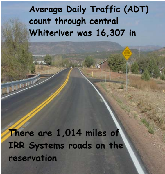
Figure 7. Typical high speed State route through Reservations.
