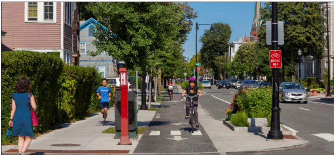
Figure 2. Image. Western Avenue Reconstruction Project with sidewalk-level separated bicycle lane and curb extensions.
