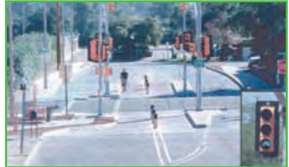
The second system, the TOCAN (TwO CAN) was installed at an intersection frequented by both pedestrians and bicyclists. The “smart” traffic signal lengthens the crossing time when cameras detect bicycles and pedestrians in the same crossing. The ease of activation — just riding up to the stop bar — is a convenience for bicyclists. The signal was implemented on a budget of \$175,000.
