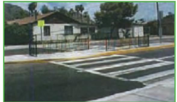
A staggered crosswalk installed for the program.
