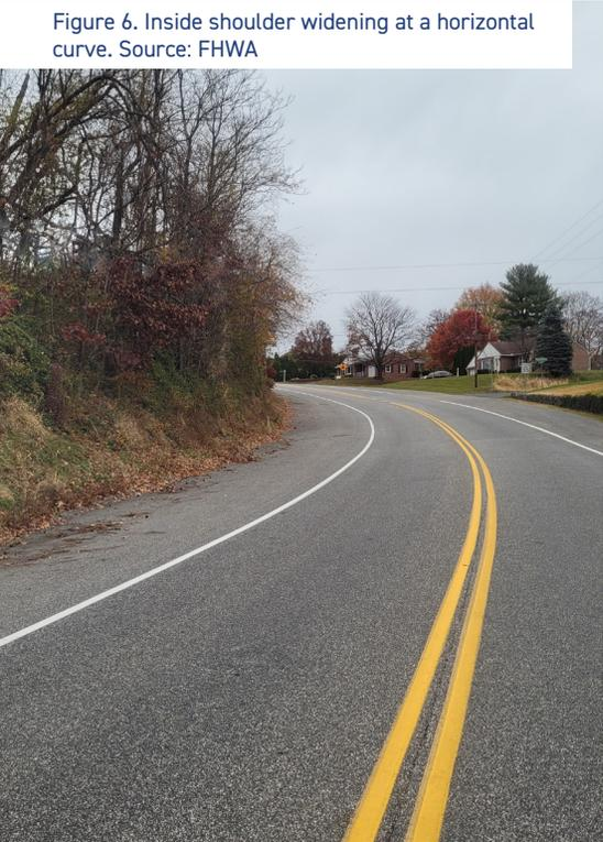
Figure 6. Inside shoulder widening at a horizontal curve. Source: FHWA
