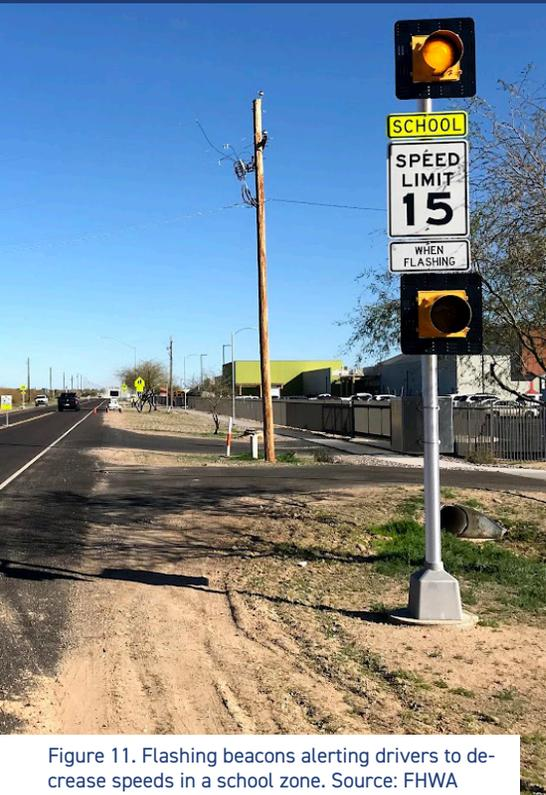
Figure 11. Flashing beacons alerting drivers to decrease speeds in a school zone. Source: FHWA
