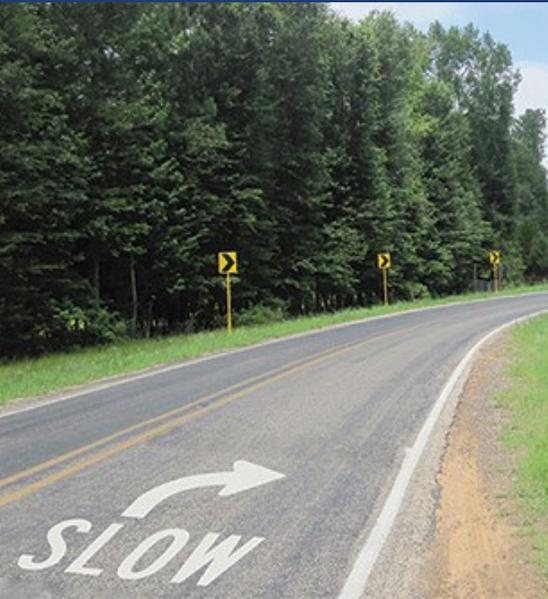
Figure 5. Curve delineation enhancements may include in-lane curve warning pavement markings and chevron signs with retroreflective strips on sign posts. Source: FHWA
