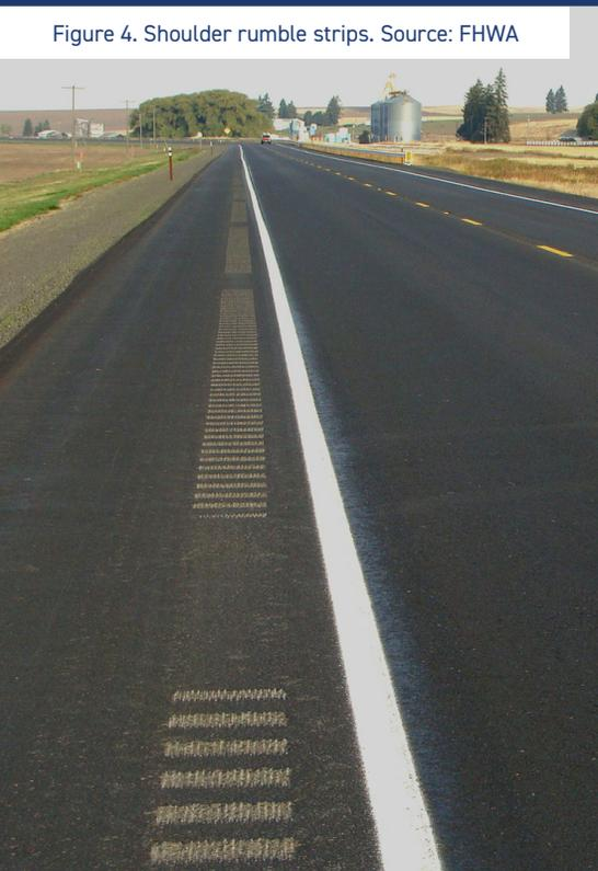
Figure 4. Shoulder rumble strips. Source: FHWA
