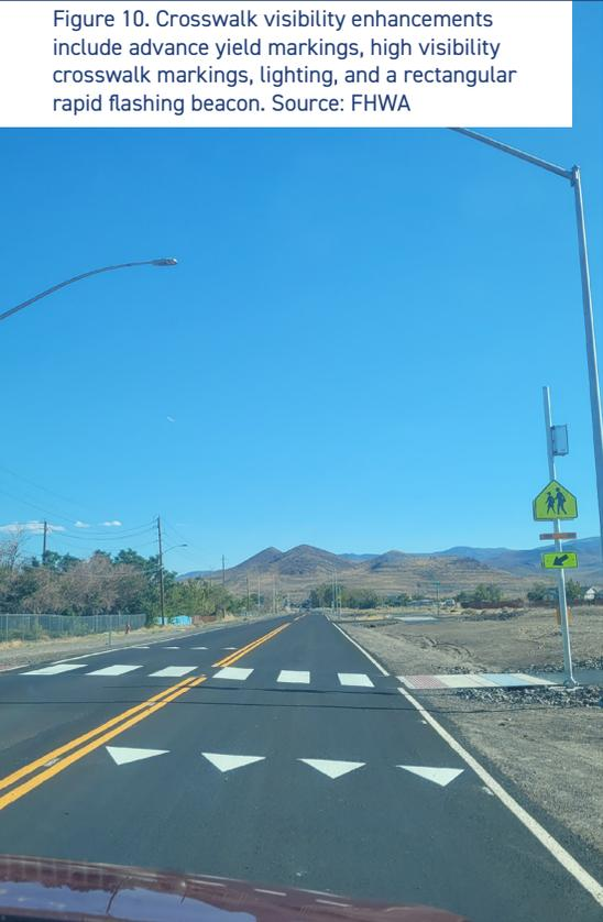
Figure 10. Crosswalk visibility enhancements include advance yield markings, high visibility crosswalk markings, lighting, and a rectangular rapid flashing beacon. Source: FHWA
