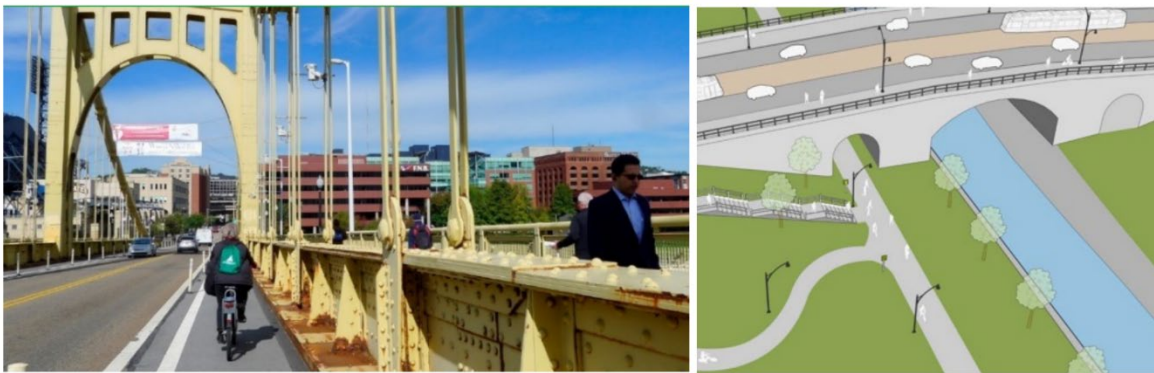
Bridge rehabilitation projects present opportunities to improve multimodal connectivity, as shown by separated travel spaces on the Roberto Clemente Bridge in Pittsburgh, PA, and design concepts linking pedestrian and bicycle routes with on-bridge facilities. Source: Reproduced from Chang et al. (2025). Left image source: Toole Design; right image source: FHWA. See endnote 2 for full citation.
