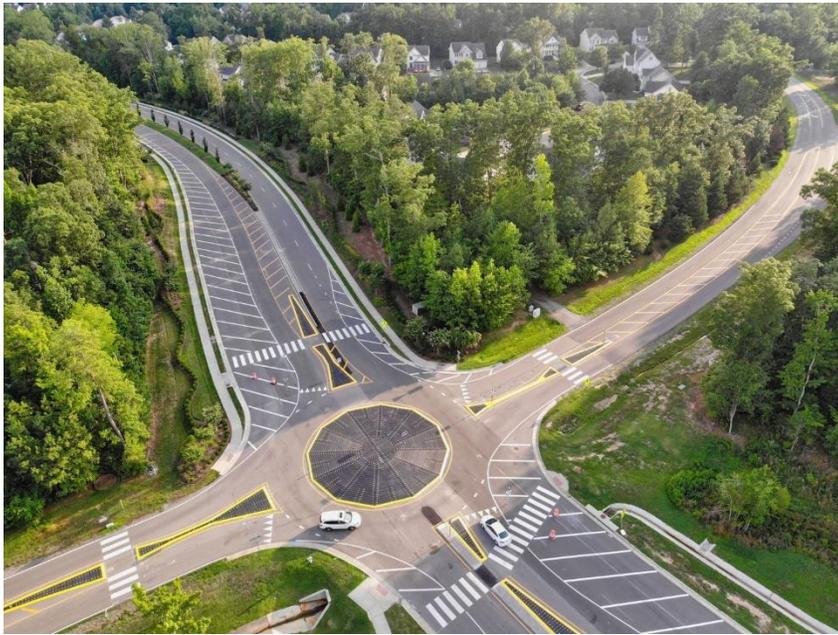
*Figure 8: An overhead look at the completed modular roundabout at Otterdale Rd/Hampton Park Dr. (Source: VDOT)*
