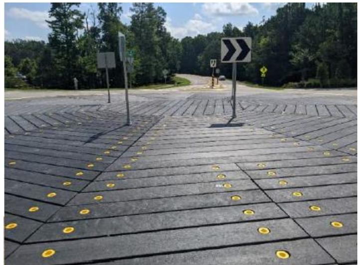
Figure 9: Modular plastic panels in the roundabout central hub. (Source: VDOT)
