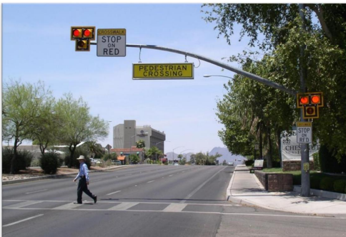
Figure 4. Example of a Pedestrian Hybrid Beacon (HAWK) treatment in Tucson, AZ, USA. 16
