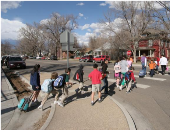
Figure 2. Curb Extension. Source: www.pedbikeimages.org/Dan Burden
