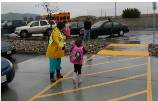
Figure 3. Raised crosswalk through school parking lot. Source: Alta Planning + Design
