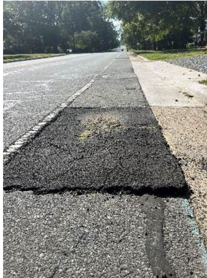
Source: BTS-10 project team
