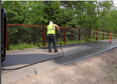
Figure 15-4: Fog Sealing a Shared Use Path
